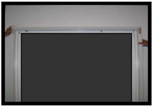
5. (FACE FIT ONLY) After securing the upper left and right corners of the frame, make sure header is STRAIGHT across the top of the window and then secure ALL support brackets onto the header frame only. After all support brackets are secured to the header frame, ensure that the header frame is STRAIGHT and secure support brackets to the wall.
