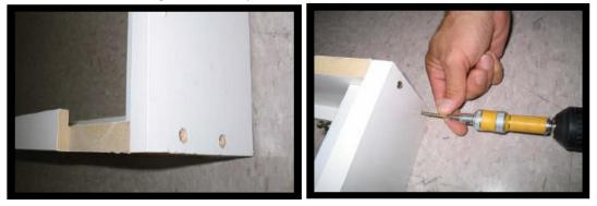
4. Place and position the assembled frame EVENLY around the window opening. Screw ONLY the upper left and right corners of the side box frame to the wall or window recess
